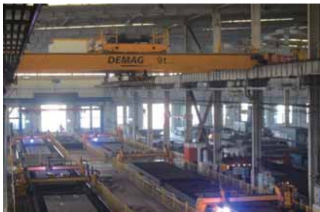
Photo: Fully-intelligent Unmanned Precision Cutting Production Line 圖：全智能無人高精度切割生產綫
